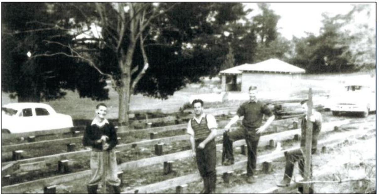
Construction Jnr Farmers Hall 1956 with Presidents Room behind.
