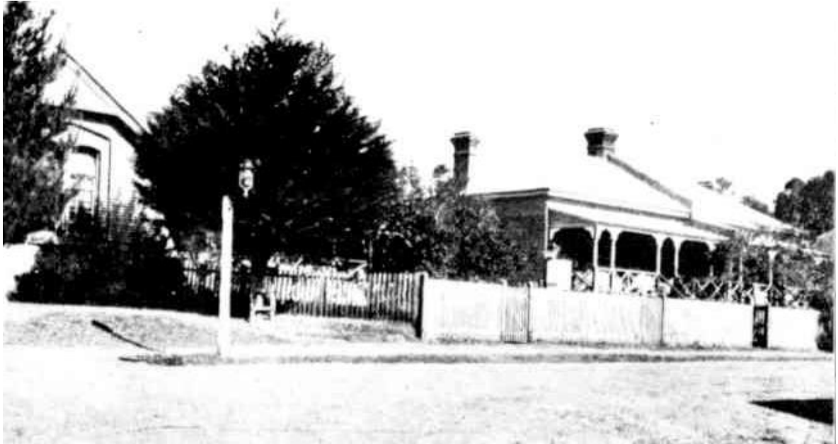
Showing the Police Quarters on the right and a glimpse of the Court House on the left
