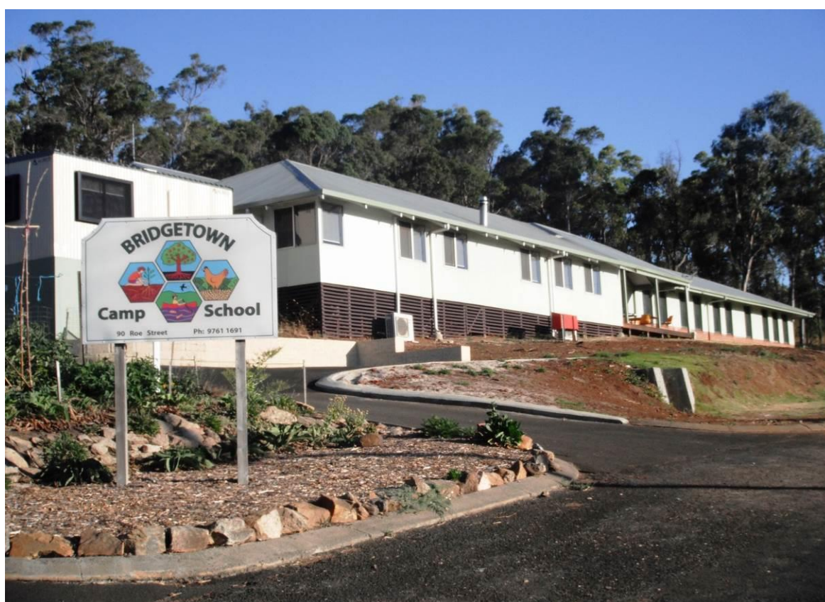
The central and southern wings of the Old Bridgetown Hospital (Camp School)
