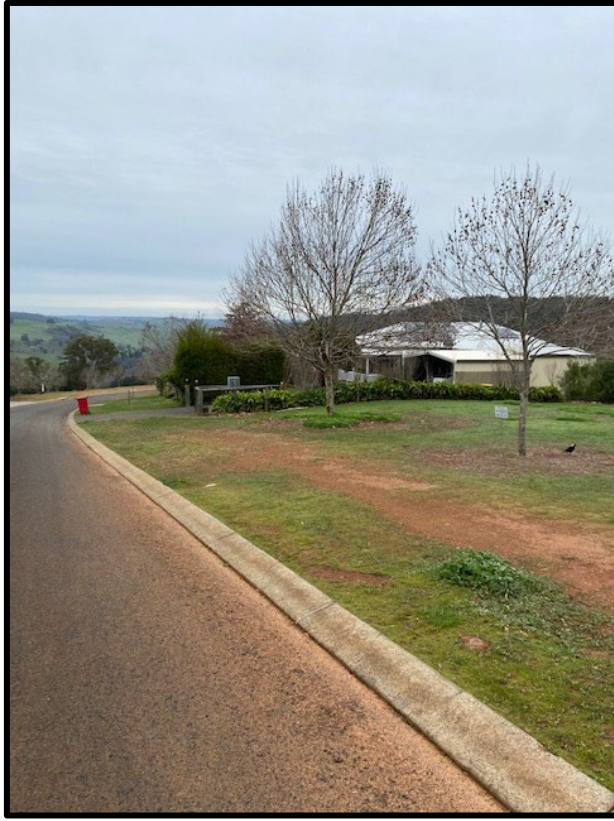
Established dwelling at 6 Riverview Close that meets the compliant setback of 12 metres
