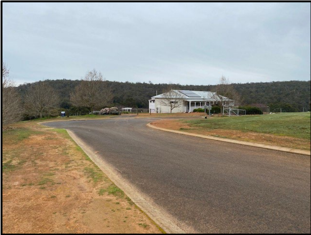
Established Dwelling at 14 Riverview Close – Located at the end of the cul-de-sac
