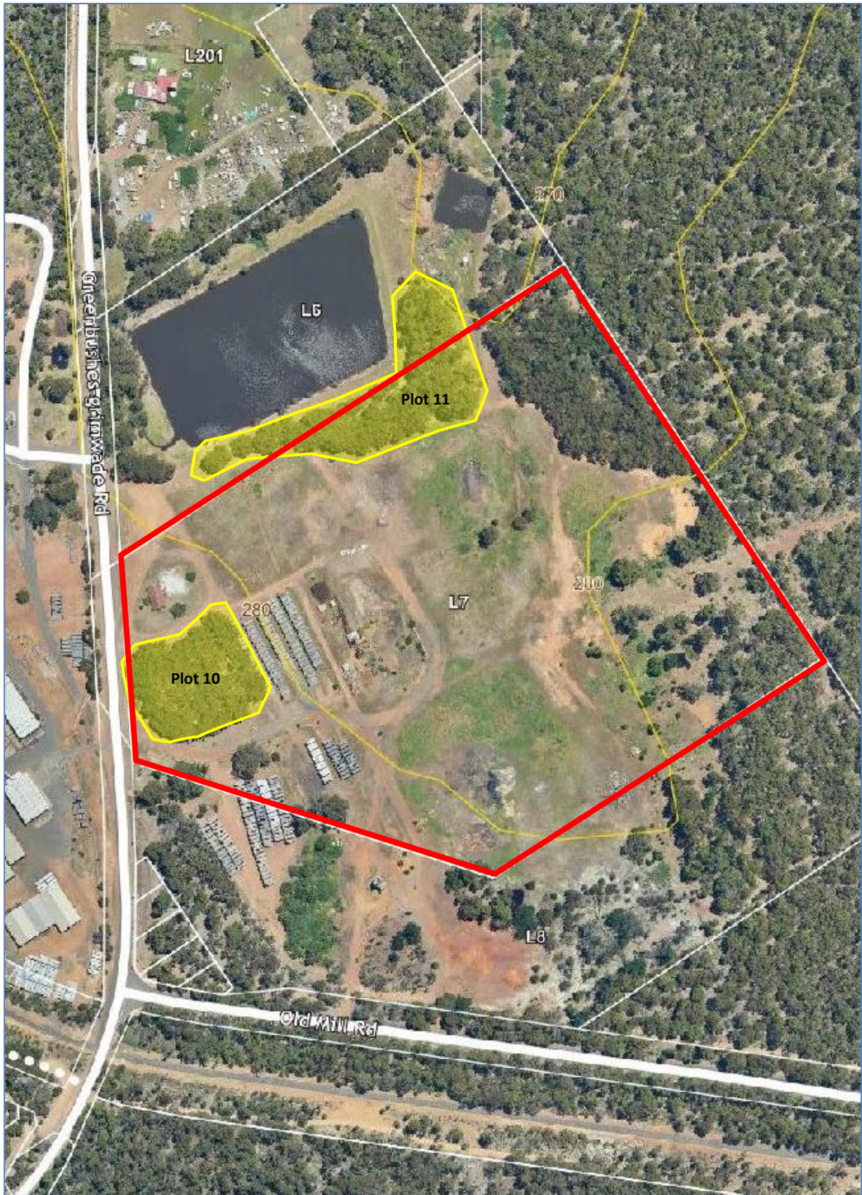
Figure 4 – Cleared Areas within Plots 10 and 11
