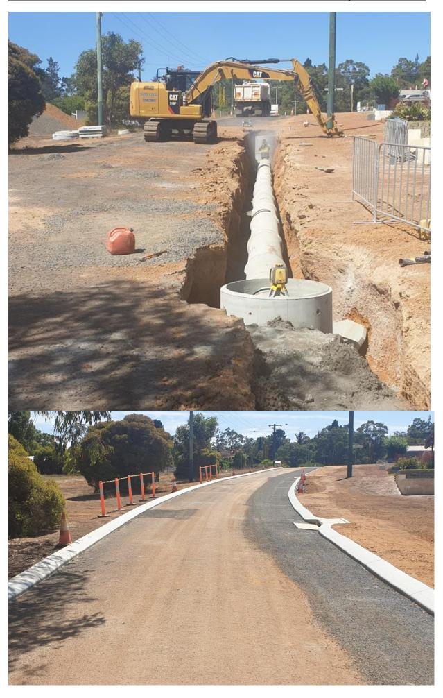
**Dairy Lane** – Works to improve drainage on Dairy Lane were completed in October. This included upgrading the existing gravel pavement to asphalt and installation of kerbing to direct stormwater. This project was completed under budget.
