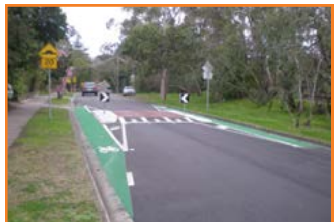
One-way slow point with bicycle-bypass facilities 3
