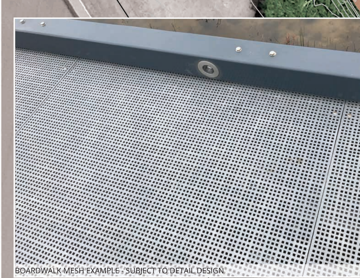
BOARDWALK MESH EXAMPLE - SUBJECT TO DETAIL DESIGN
