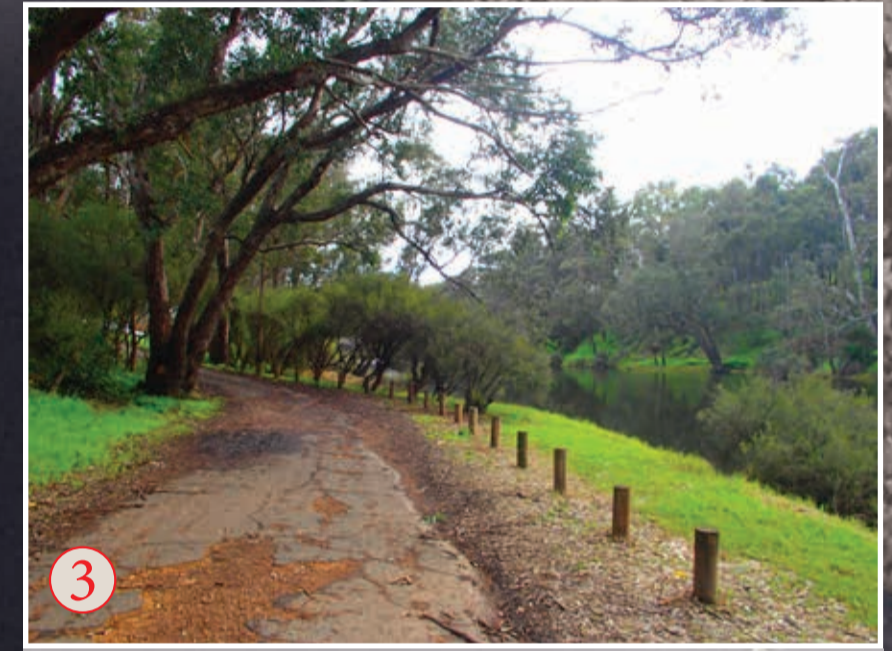
EXISTING SITE CONDITION
