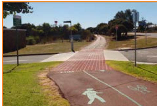
Shared path with priority over minor road
