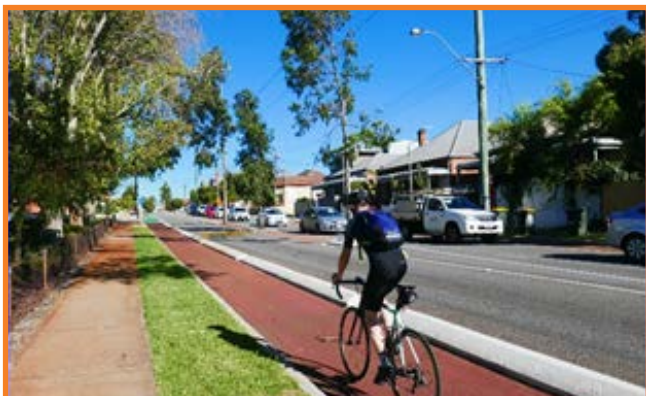
Bike lane protected by concrete kerb
