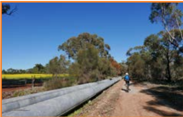
Trail within utility corridor
