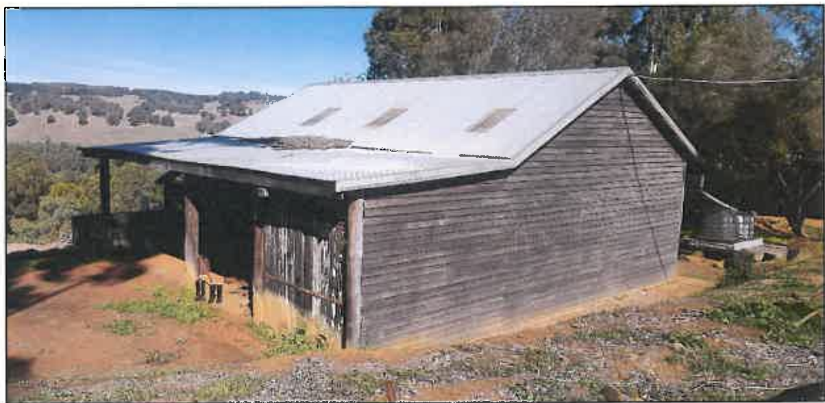
Existing Barn at Lot 125 (22) Bovell Street, Bridgetown
