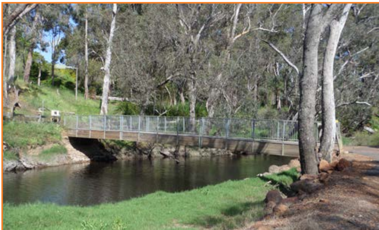
Figure 4.10 This footbridge in Bridgetown enables pedestrians and cyclists to experience both sides of the Blackwood River.
