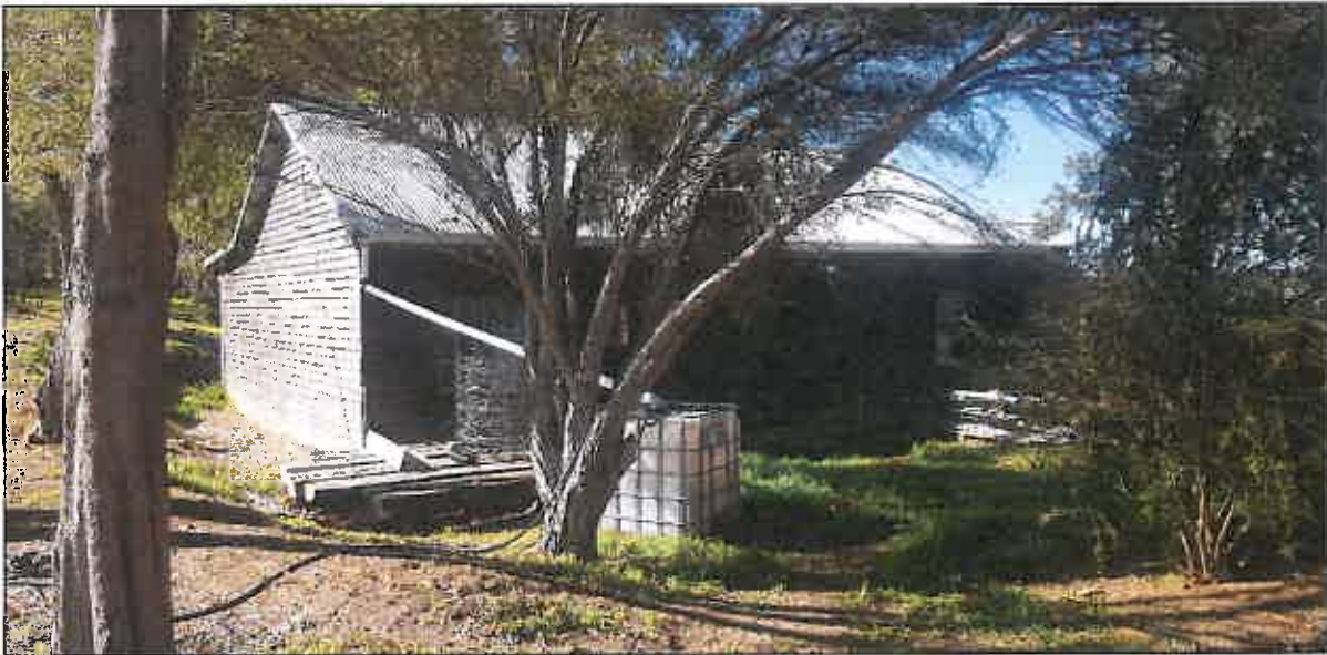
Existing Barn at Lot 125 (22) Bovell Street, Bridgetown
