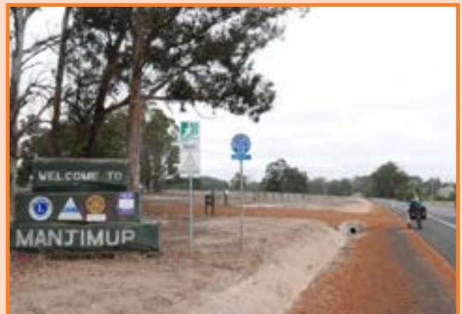
Figure 4.23 Shoulder widening along Muirs Highway
