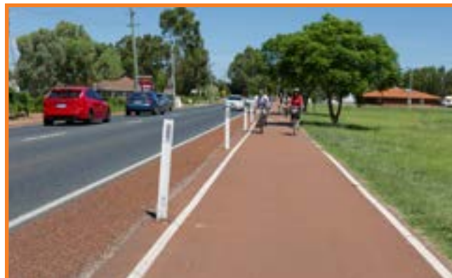
Bi-directional bike lane separated with bollards
