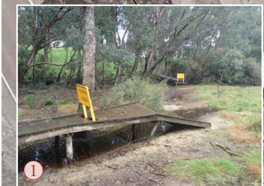
EXISTING SITE CONDITION
