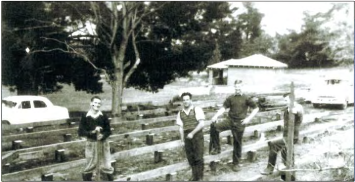
Construction Jnr Farmers Hall 1961 with Presidents Room behind.
