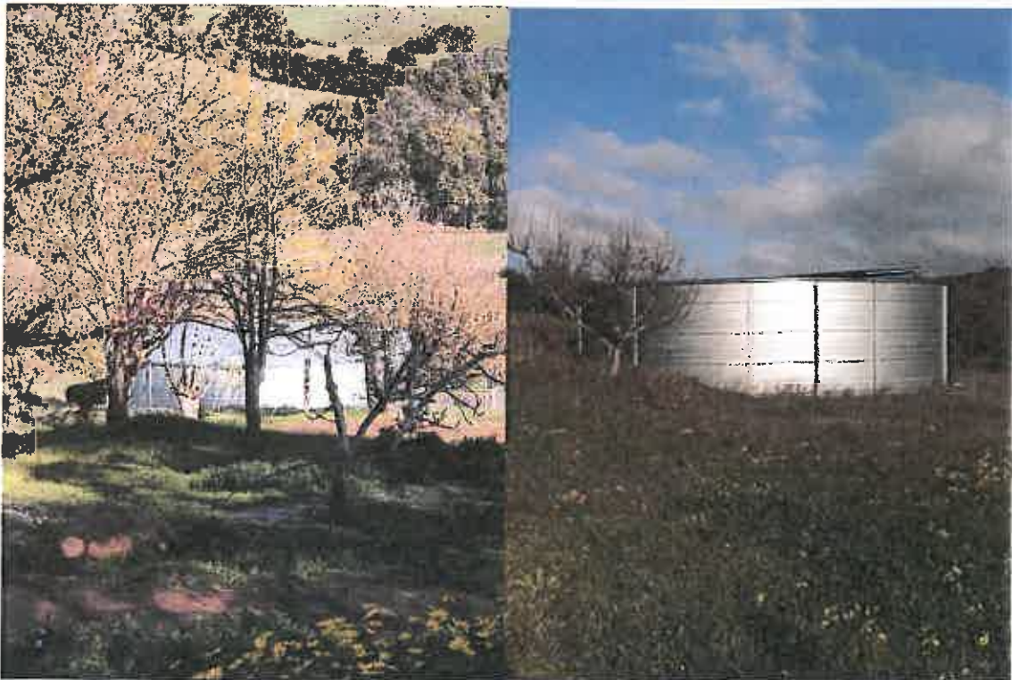
Left photo : View from our bedroom window showing sides and top of water tank. A similar outlook is also visible from several other house rooms. Right photo shows proximity to fence line and that no attempt to screen the tank or reduce the glare from its reflective surfaces despite being installed about 3 years ago. Both photos show this tank is visible across the valley.
