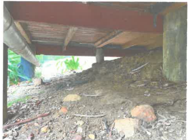
Typical sub-floor frame
