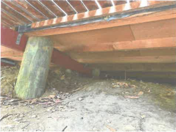
Typical sub-floor frame
