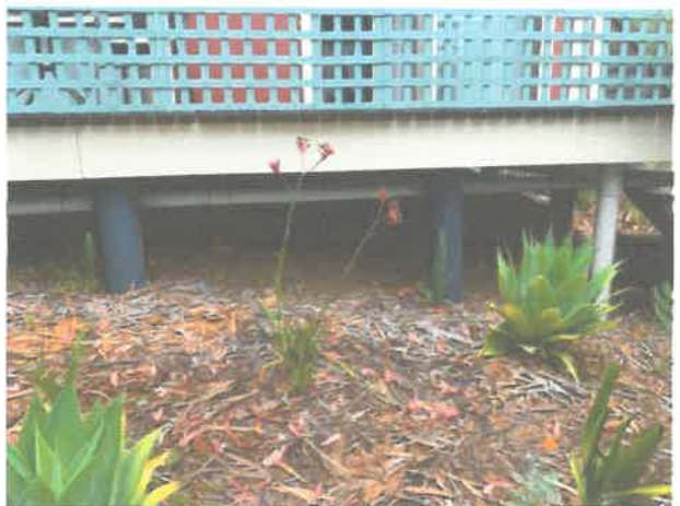
Front verandah deck
