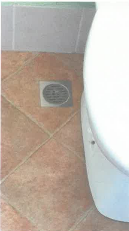
Floor waste installed
