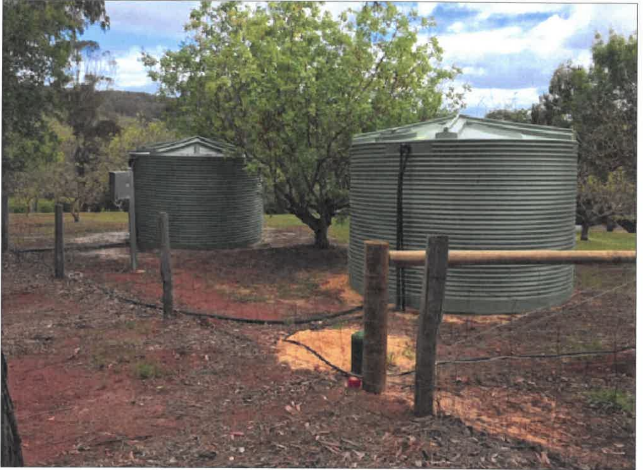
Water Tanks at 15 Mottram Street, Bridgetown
