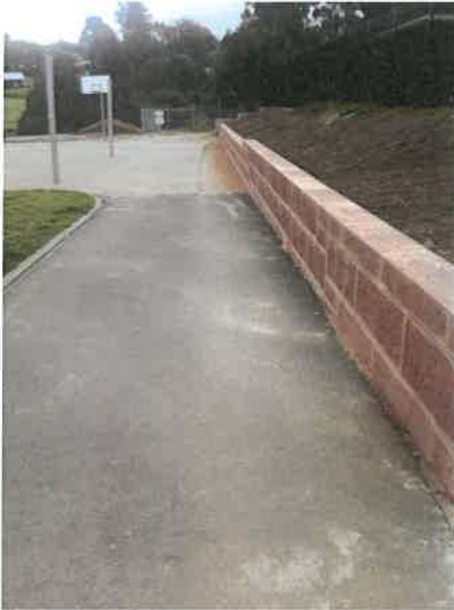
Existing path running along the base of a portion of the new retaining wall looking north towards the basketball court and gas chlorine storage facility
