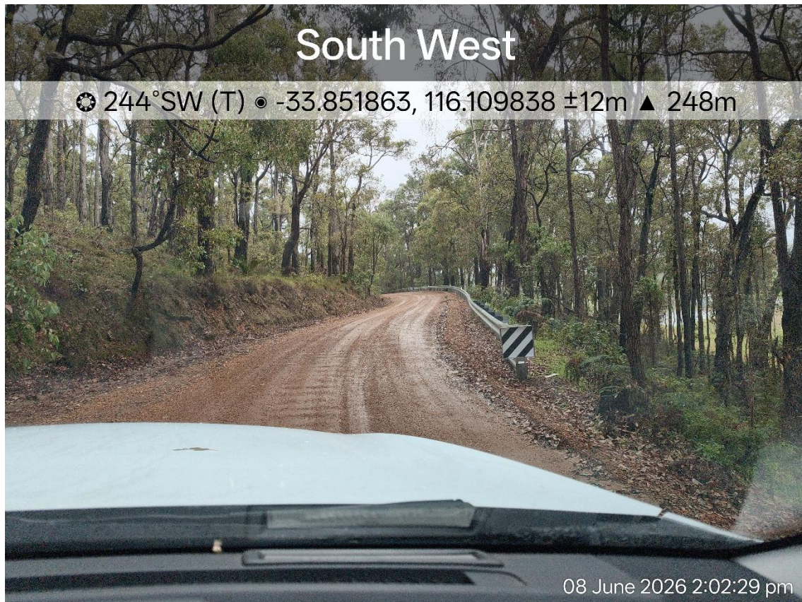
Figure 27 – Catterick Road at SLK 2.41 (Narrow Unsealed Section)
