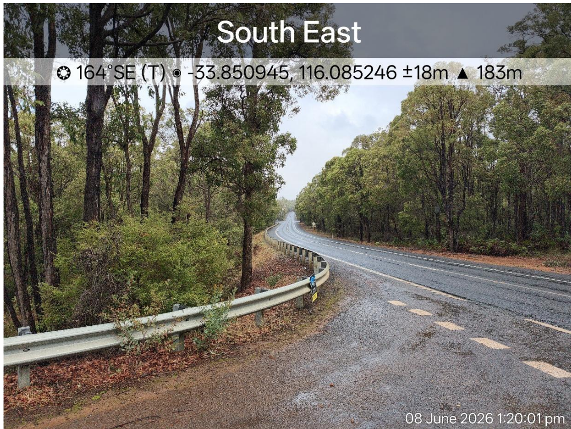
Figure 24 – Catterick Road approaching South Western Highway (looking south east)
