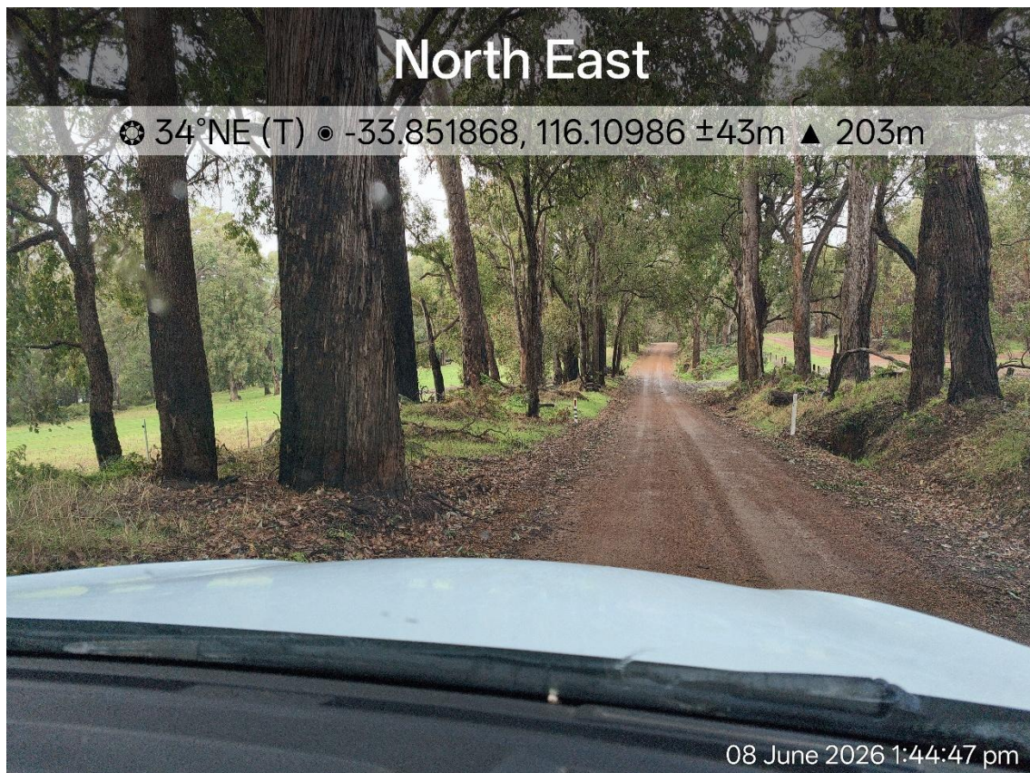
Figure 28 – Catterick Road at SLK 2.42 (Narrow Unsealed Section)
