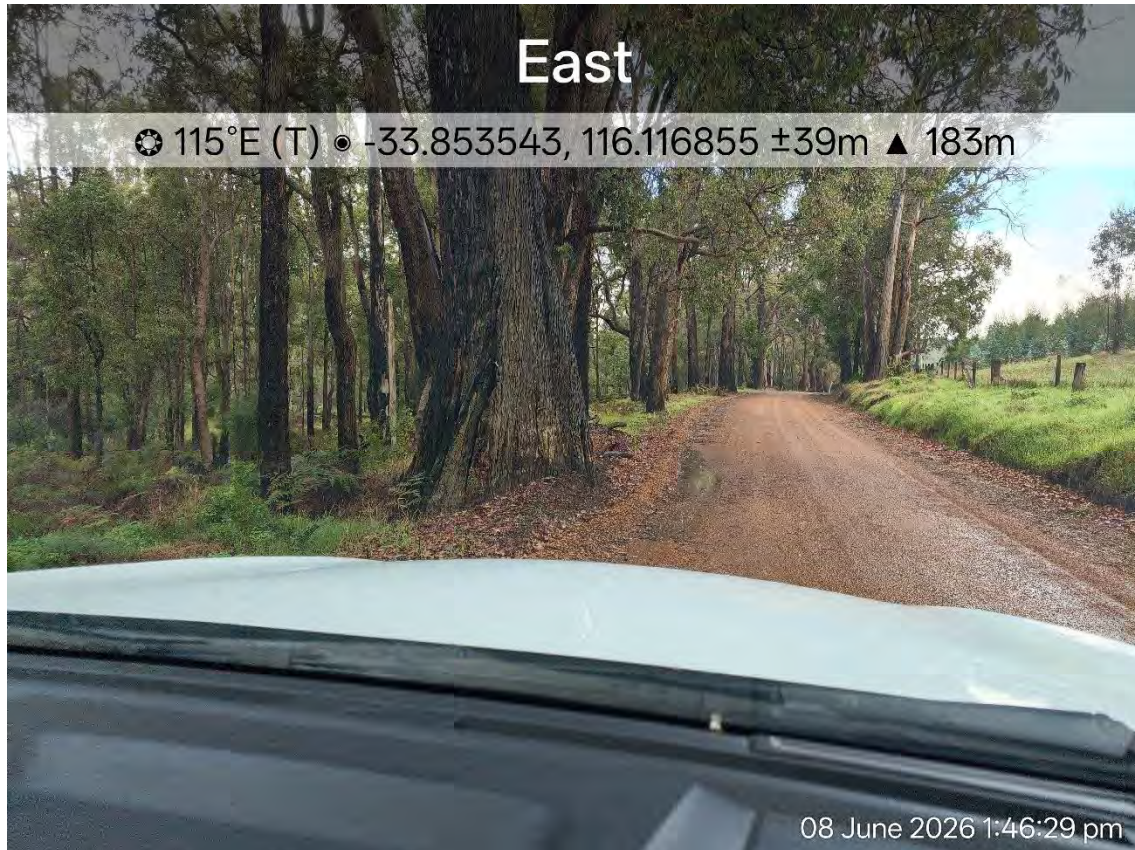
Figure 29 – Catterick Road at SLK 3.21 (Narrow Unsealed Section)
