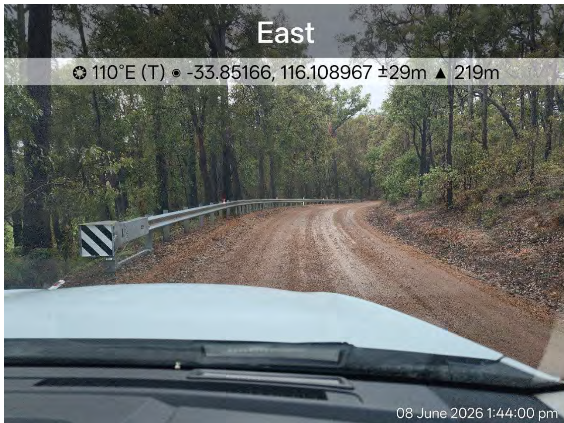
Figure 26 – Catterick Road at SLK 2.31 (Narrow Unsealed Section)
