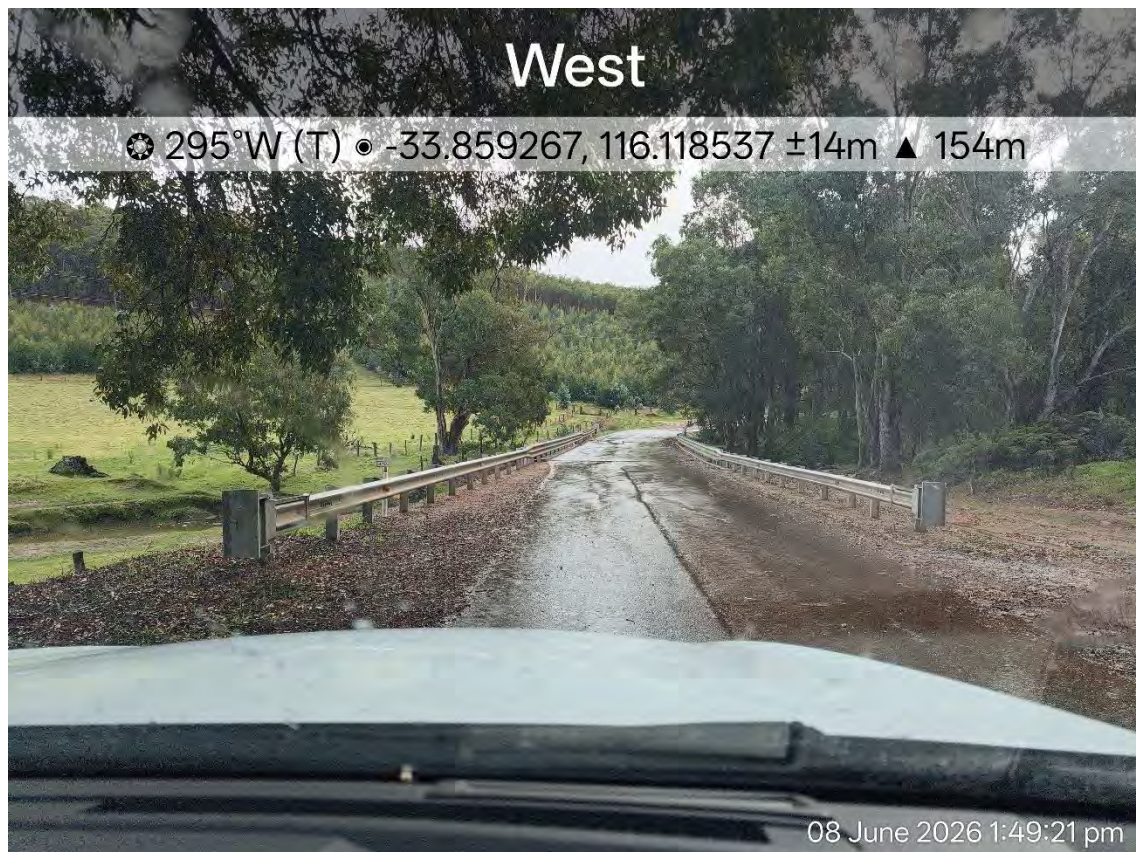
Figure 32 – Catterick Road at SLK 3.87 (Existing Bridge crossing the Hester Brook Creek)
