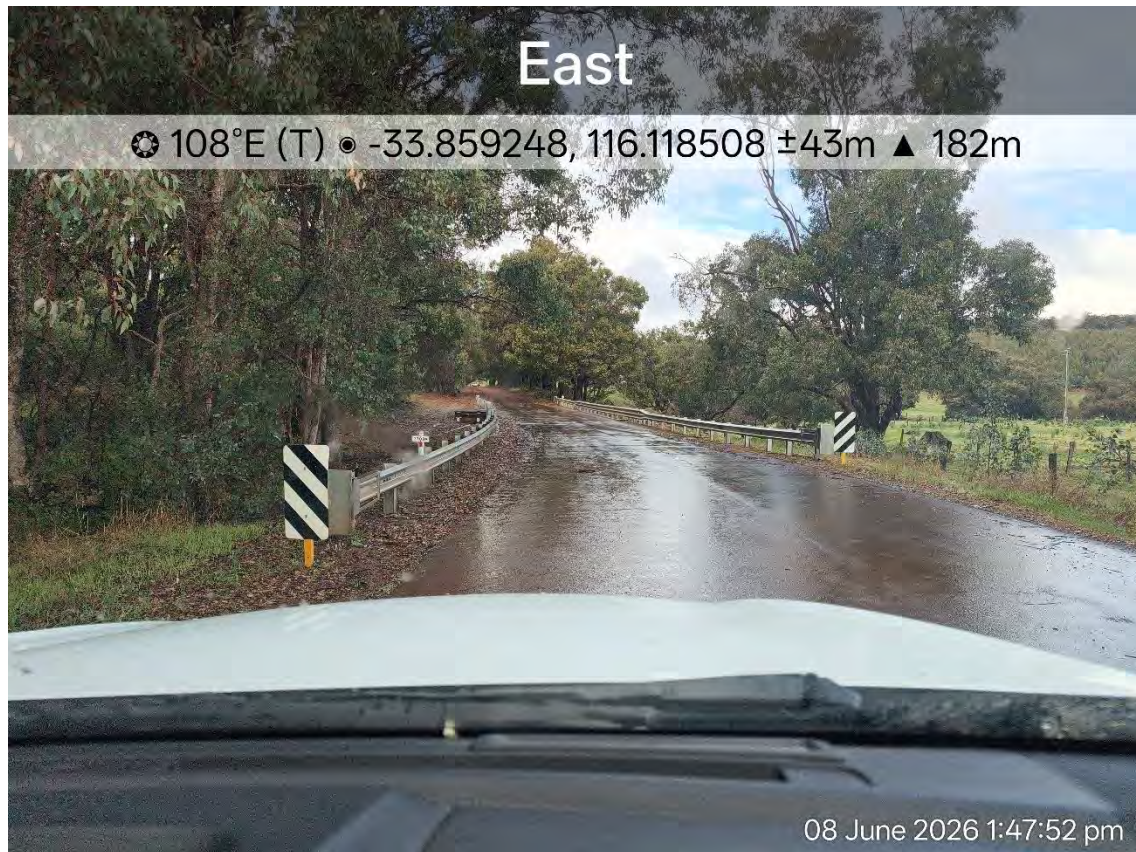
Figure 31 – Catterick Road at SLK 3.74 (Existing Bridge crossing the Hester Brook Creek)
