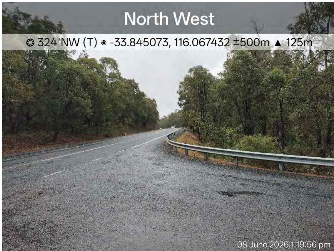
Figure 25 – Catterick Road approaching South Western Highway (looking north west)
