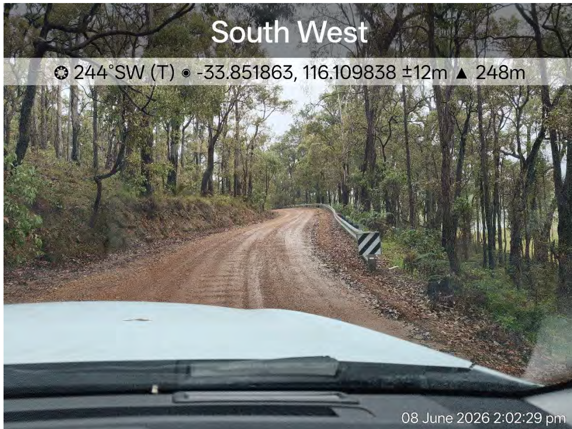
Figure 27 – Catterick Road at SLK 2.41 (Narrow Unsealed Section)
